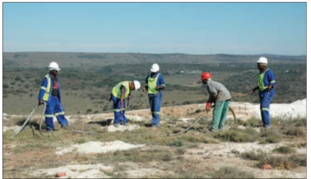
Workers carefully set up the equipment.
