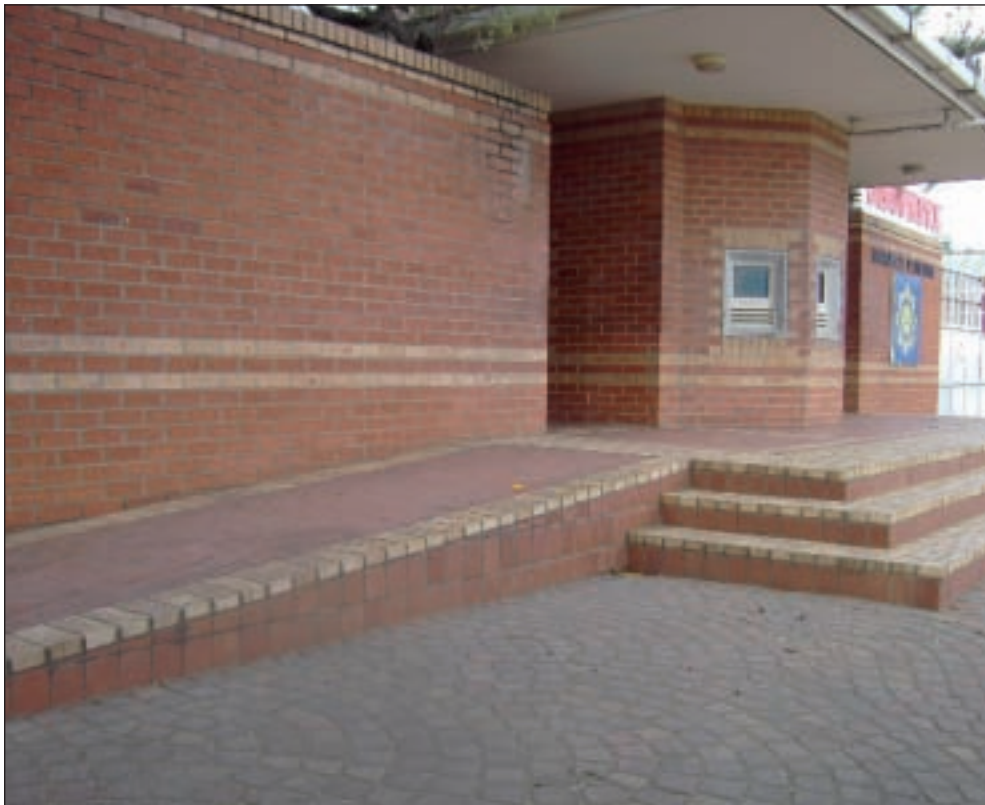
ACCESS GRANTED... A wheelchair ramp outside the police station. Photo: Babongile Zulu
